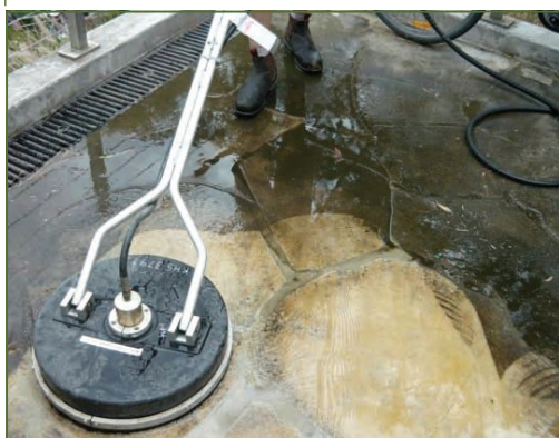
Cleaning and preparing the sandstone.
