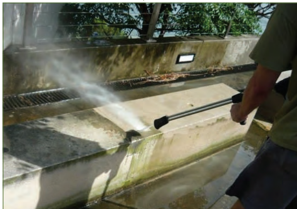
Cleaning and preparing the sandstone.
